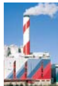
Waste incineration plants.
